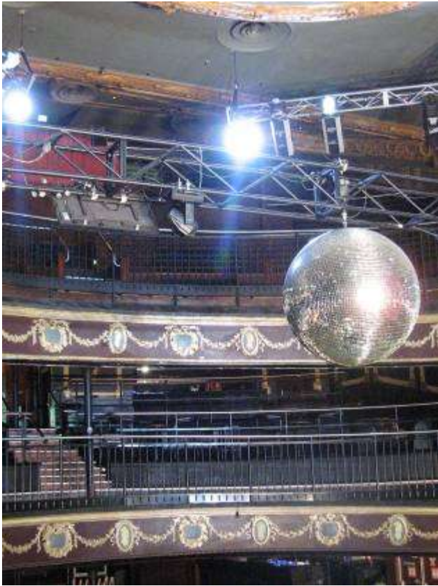
Balcony balustrades with 1916 plaster decoration
