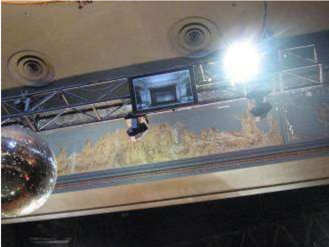
Proscenium decoration (re-installed)
