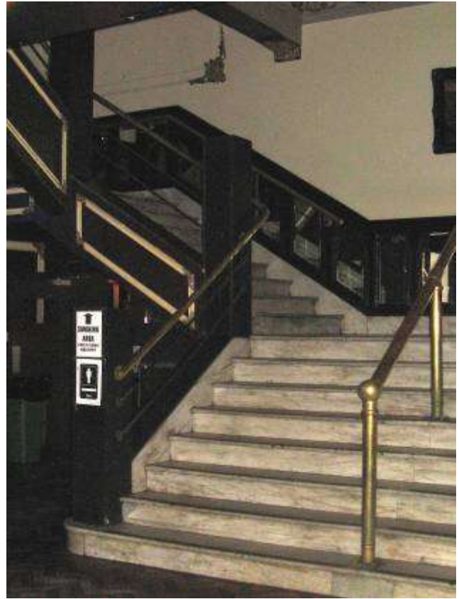
The main stairs of marble (1916)
